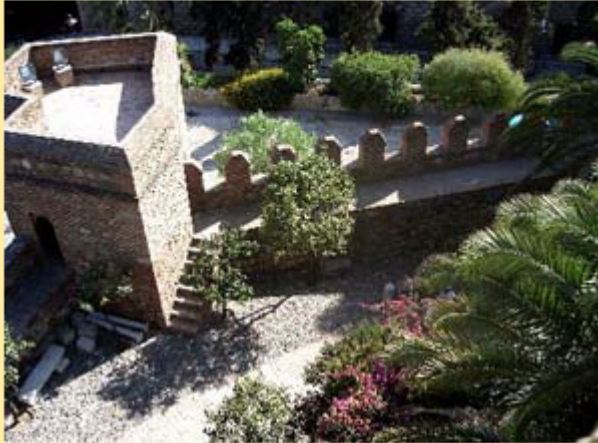
The walls of the 'Alcazaba' in Málaga.
